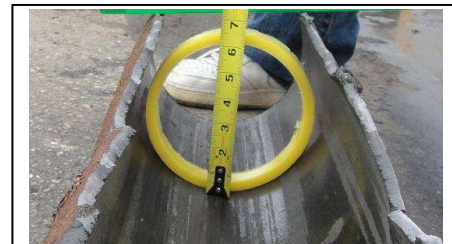
[Fig. 7] Cut open cast iron pipe and PE pipe
